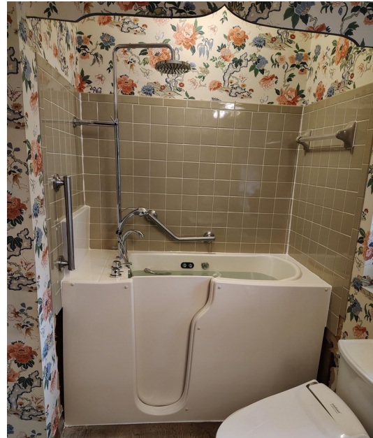
Walk-in tub fitted into an existing traditional bathroom.
