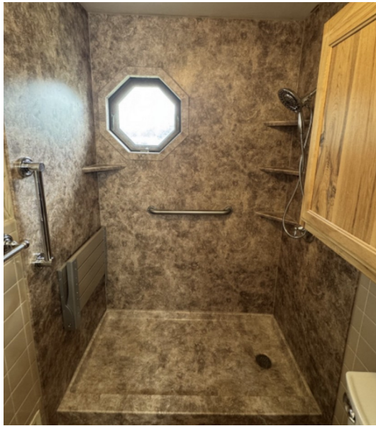
Finished shower with grab bars and fold-down seating.
