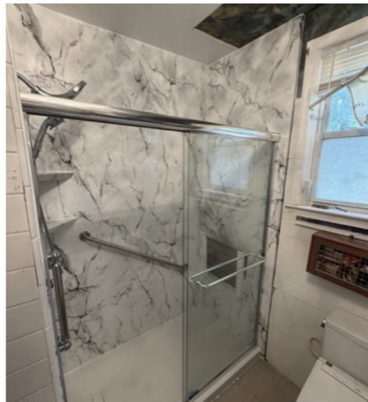
Finished accessible shower with glass enclosure.
