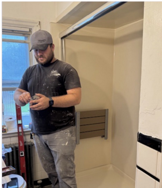
Real installation work in progress.
